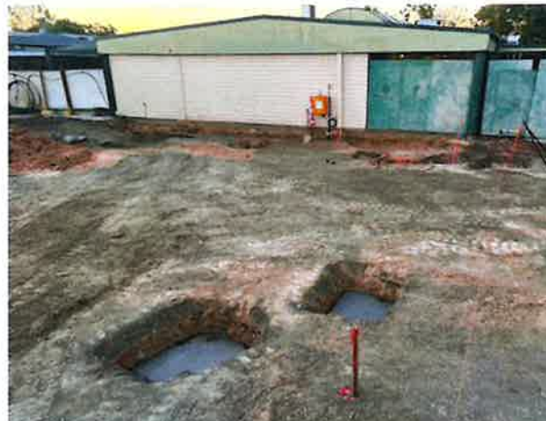
Pad Footings Poured for Covered Play Area
